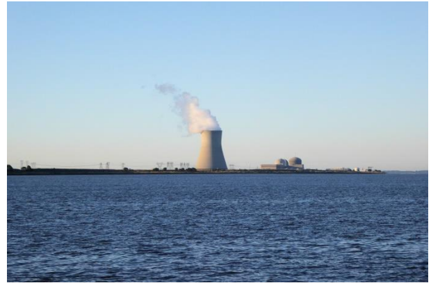
The Salem Nuclear Power Plant
