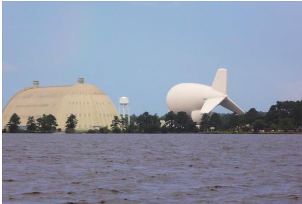
The blimp hangar on the Pasquotank River
