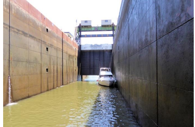
Our travelling companions behind us in the 40' lift lock
