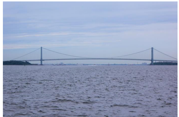
The Verrazano Bridge leading into New York Harbor
