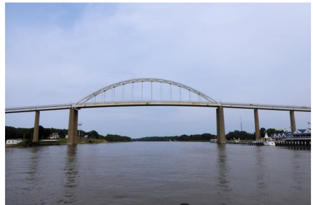
One of several bridges over the C&D Canal
