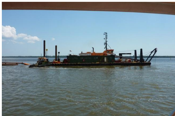
Dredge on the ICW near Kings Bay Submarine Base
