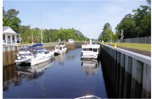
The South Mills Lock on the Dismal Swamp Canal
