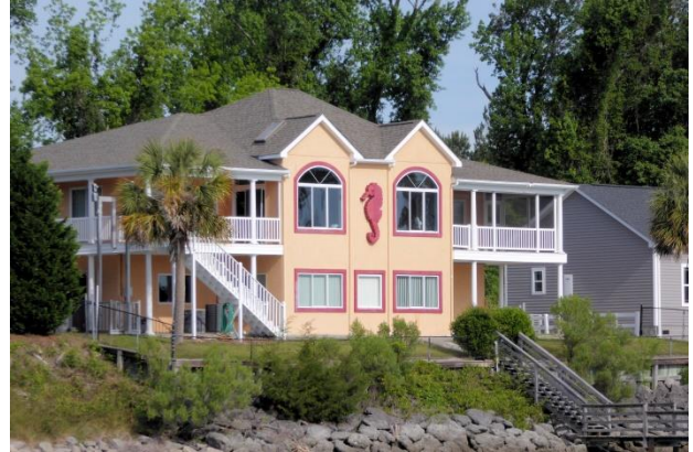
One of the nice homes on Adams Creek
