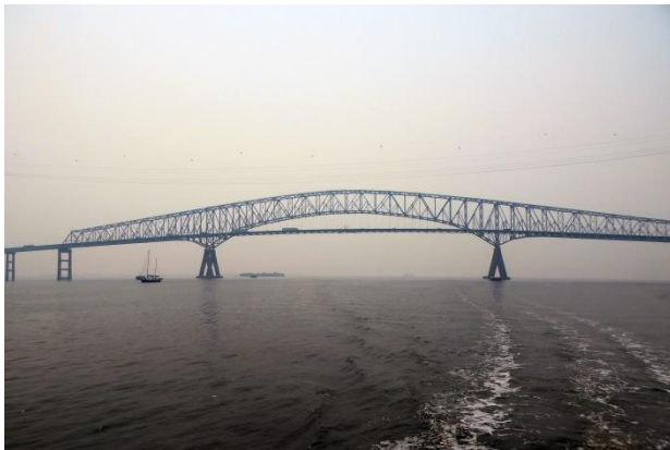
The Francis Scott Key Bridge on the way to Baltimore, MD
