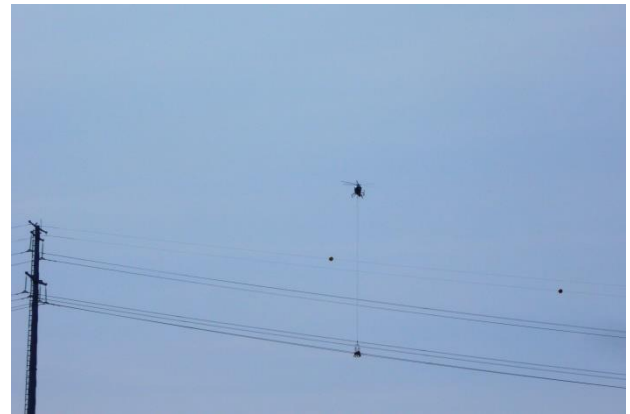
Workers suspended from a helicopter, working on the lines
