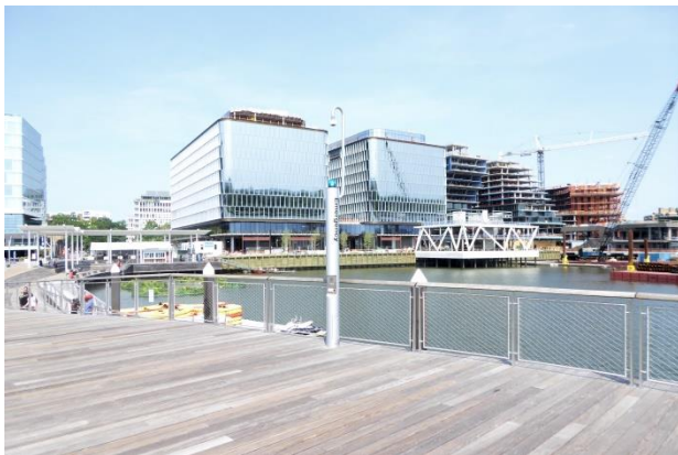
Looking south from the Recreation Pier
