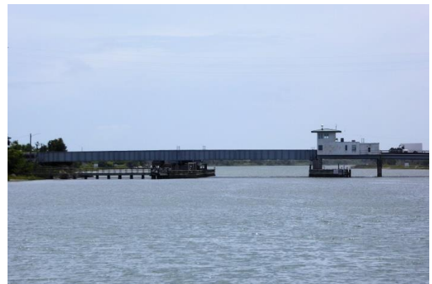
Onslow Beach Swing Bridge
