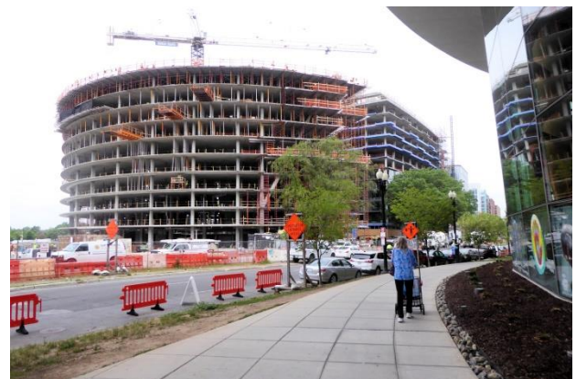
Construction along the Wharf area
