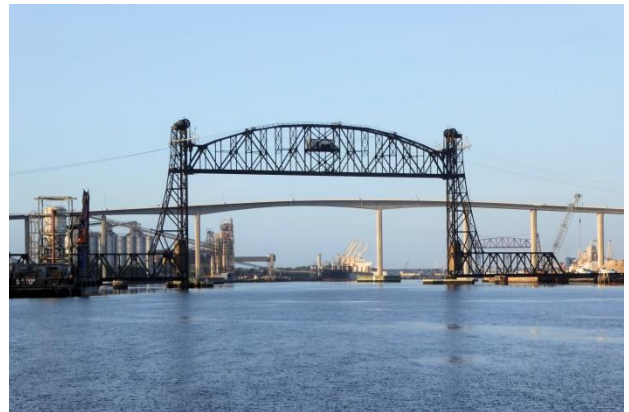
One of the lift bridges we were concerned about
