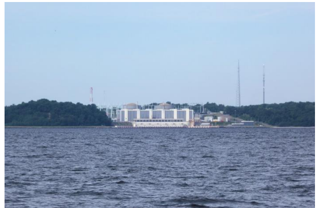
The Calvert Cliffs Nuclear Generating Plant
