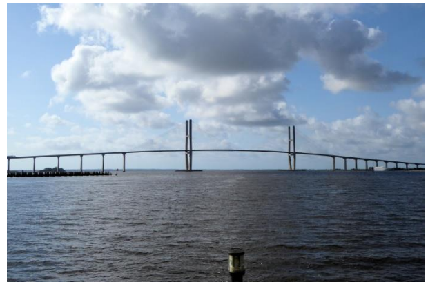
The Sidney Lanier Bridge near Brunswick, GA
