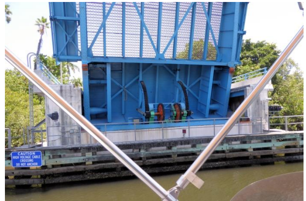
The seldom seen underside of a drawbridge
