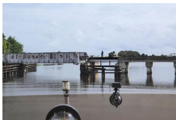
The Moore Haven Railroad Bridge
