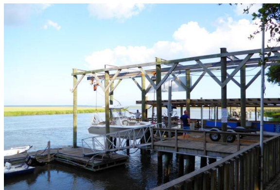
No ramp here, this is how they launch boats
