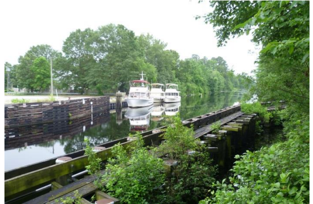
Waiting for the Deep Creek Lock to open
