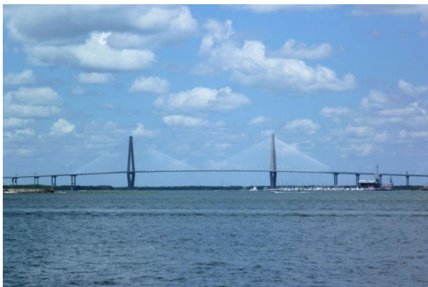
The Cooper River Bridge – we are getting close to home
