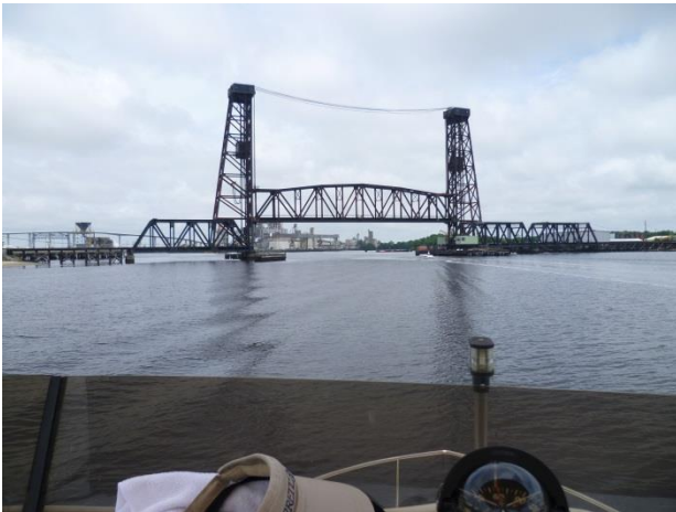
A railroad lift bridge on the ICW in Norfolk
