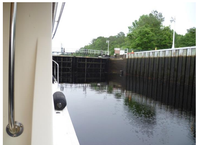
Lowered eight feet and waiting to exit the lock
