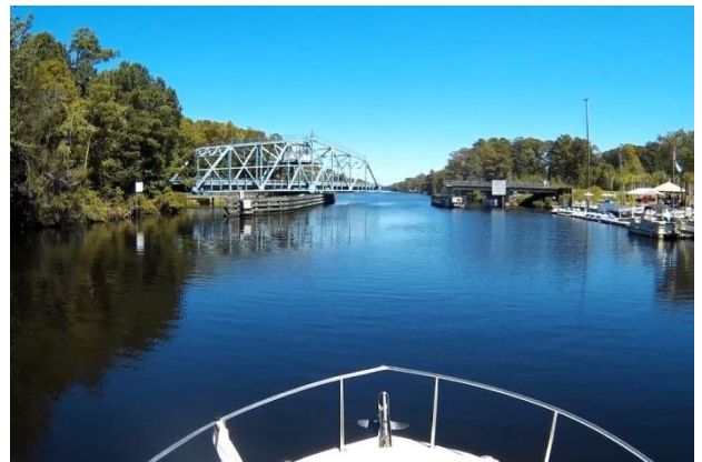
ICW Bridge opening - Socastee Swing Bridge, Socastee, SC
