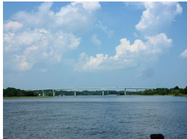
Nearing Charleston, SC - The Limehouse Bridge
