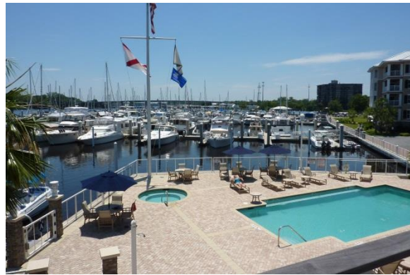
The Marina at Ortega Landing
