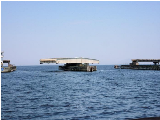
The Alligator River Swing Bridge – The Alligator River, NC
