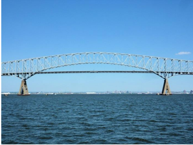
Francis Scott Key Bridge - Baltimore, MD
