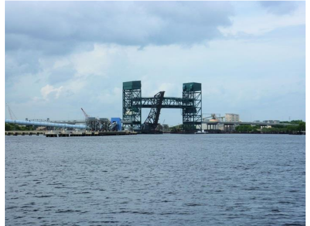
Railroad Lift Bridge, Norfolk, VA
